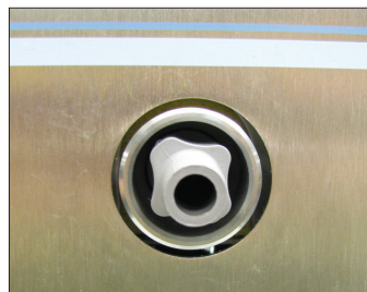
Installed Drain Fitting with Cap Removed
